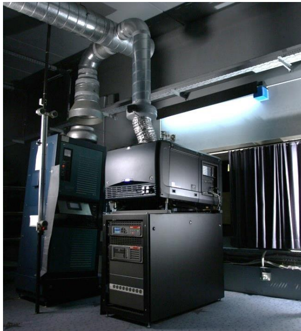
Figure 2. A projector booth with a digital and a film projector and top exhaust systems
