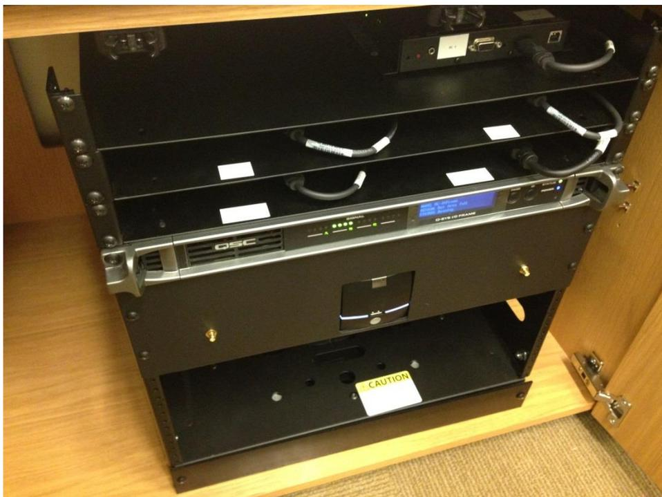
Figure 8: Example of wrong ClickShare installation: the antenna are not connected on the ClickShare rack-mounted kit
