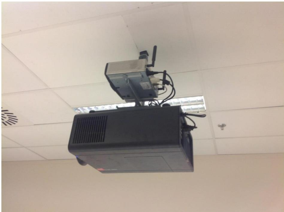
Figure 6: Example of correct ClickShare base unit installation
